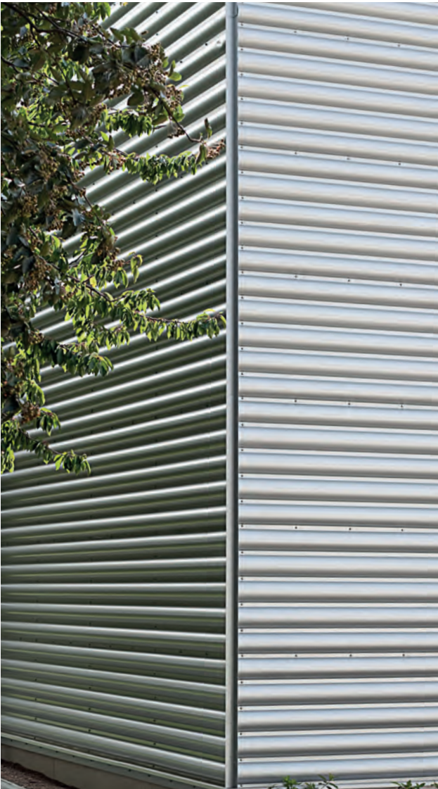
Integrated building project in South Yorkshire.
