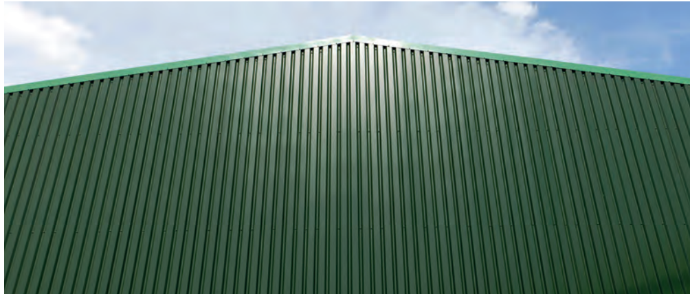
JI Shield Built-up System - West Midlands project
