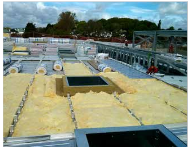
Soaker with rigid insulation in place
