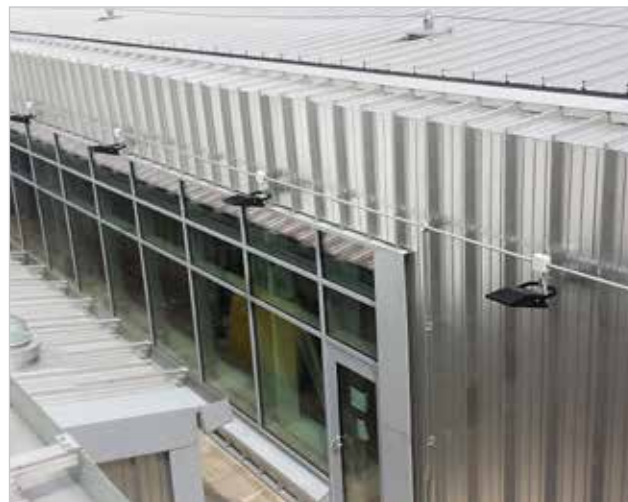
Factory pre-formed cranked sheets
