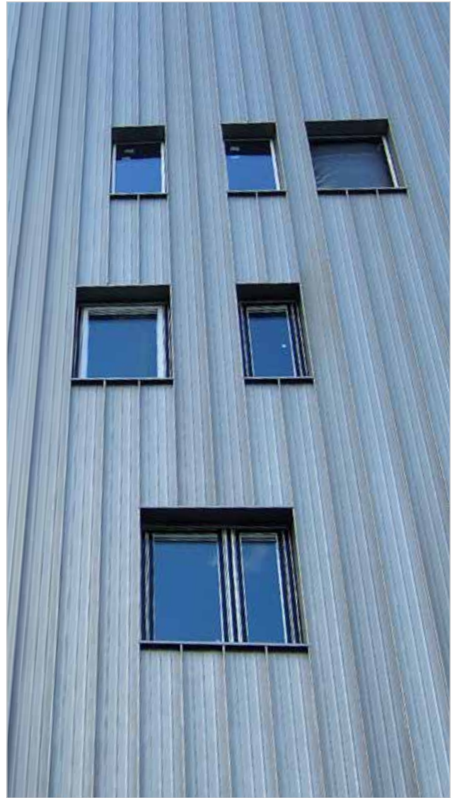
Walsall College, Shepperd Construction
