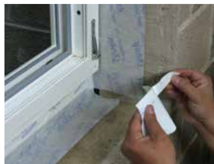
9. Remove the release paper from the back of the tape
