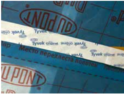
10. Seal laps with Tyvek® Tape (Tyvek® Metallised Tape should be used with DuPont™ AirGuard® Reflective)
