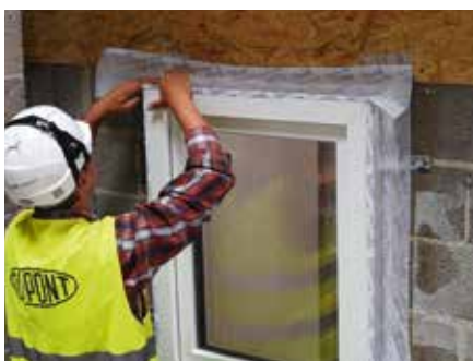
10. Complete the sealing work at the window head
