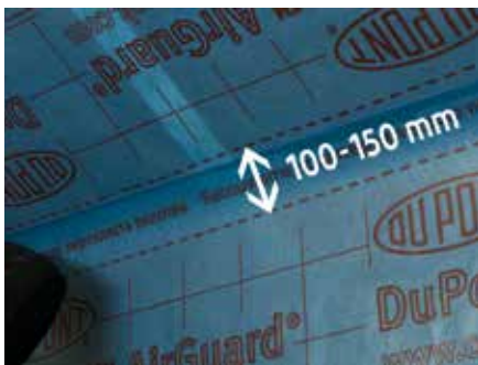
7. Apply AVCL, ensuring successive runs are adequately lapped to each other and onto adjacent wall surfaces
