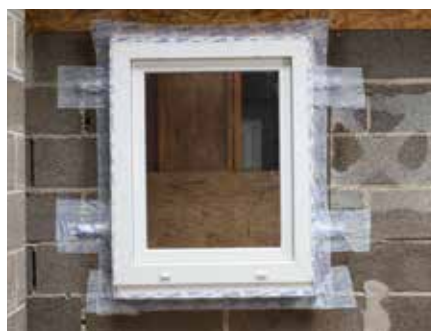
11. Tape over any exposed brackets and the sealing work is complete
