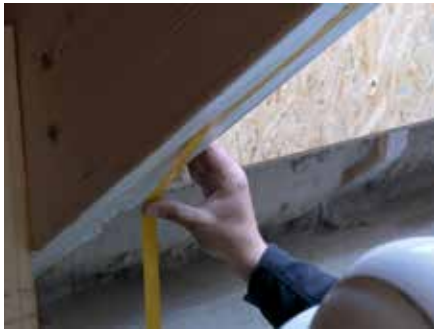
1. Apply Tyvek® Double-sided Tape (20mm) to underside of rafters
