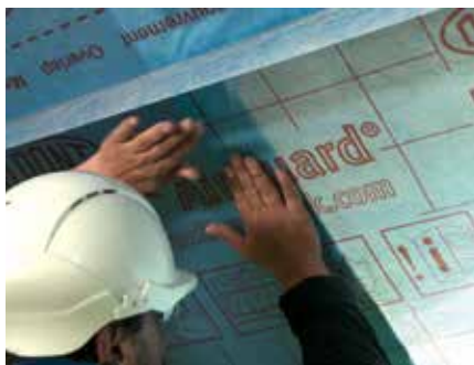
8. AVCL should be pressed firmly against tape
