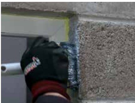
7. The primer is white on application, but will turn transparent when it cures after 1 hour approx.
