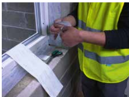
7. Fold and stick the tape to form a small corner detail...
