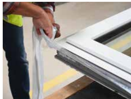
3. Form a loop on the corners: 1.5 x joint width. Seal or press together firmly
