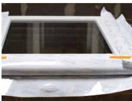
8. Fold the skirt and temporarily fix back with tape before installing the window
