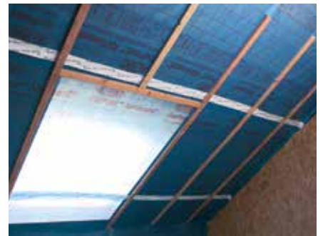
15. Battens should be suitably positioned for fixing of plasterboard lining
