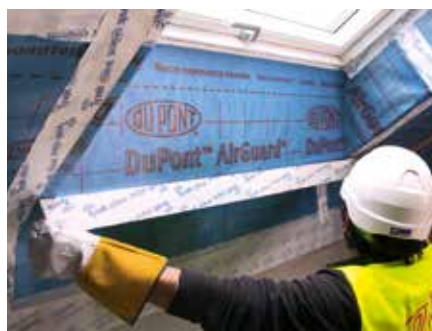
11. All cuts, laps & junctions in the membrane should be sealed with DuPont™ Tyvek® Acrylic Tape
