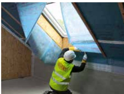
4. Cut AVCL horizontally across foot of window, in line with the reveal edge
