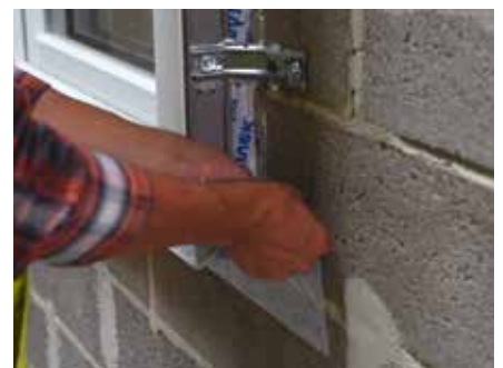
6. ... dress the tape around the detail and press into place
