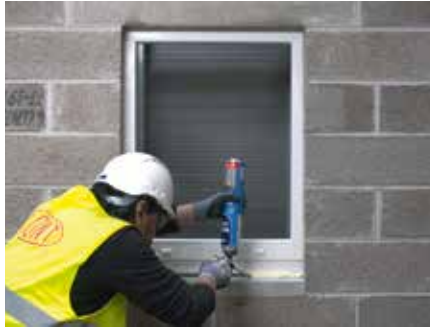
2. Shake can thoroughly and apply DuPont™ Insta Stik™ into the gaps around the window
