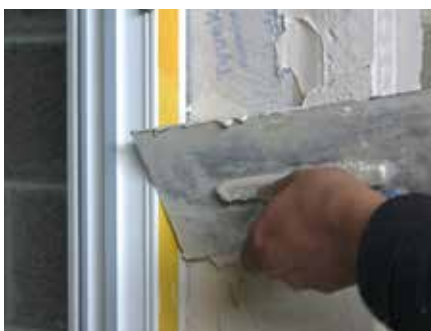
11. Tyvek® Plastering Tape provides a suitable key for the application of plaster or render
