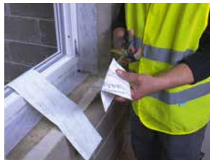
3. Cut half way along the crease
