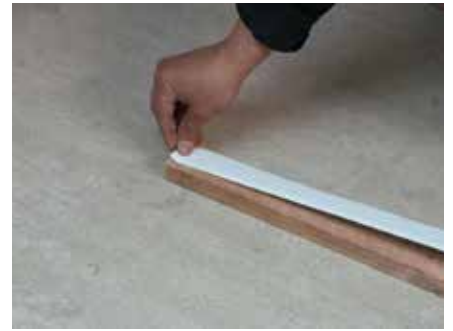
12. Apply Tyvek® Butyl tape to batten
