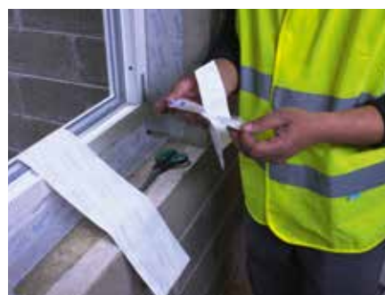
6. Remove a quarter of the release paper from the back of the tape
