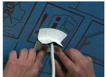
6. Press into position ensuring no gaps are present
