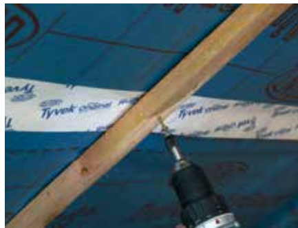
14. Press batten into position and permanently fix
