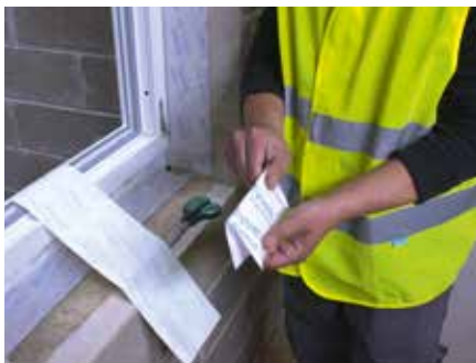
2. Internal corners can be sealed with a separate piece of Tyvek® Plastering Tape. Firstly, cut out a square of tape and fold in half
