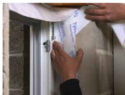
9. When the window unit is fixed into the opening remove the remaining release paper and apply Tyvek® Plastering tape on the interior side of the window. Finish as per page 36.
