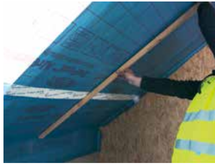
11. Measure battens prior to fixing
