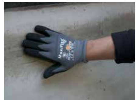
6. After an hour the primer turns transparent
