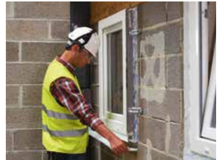
3. Position and secure the window unit and seal the external window/wall junction using Tyvek® Plastering Tape
