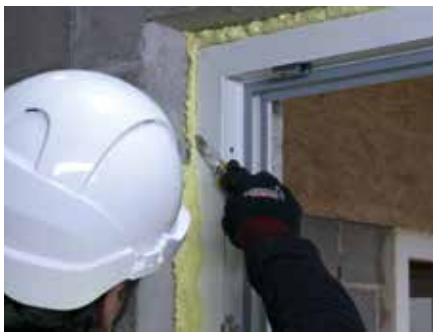
4. The spray foam will cure in around an hour and any excess can be trimmed off
