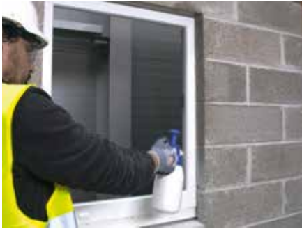
1. Spray water onto external surfaces to effect bond with DuPont™ Insta Stik™
