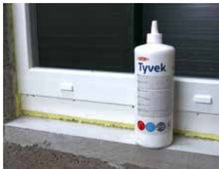
5. If the surfaces around the frame need to be stabilized Tyvek® Primer can be applied to improve adhesion for sealing tape
