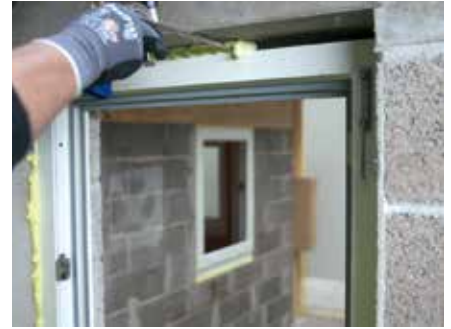
3. Repeat the process from inside the building
