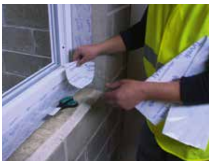
8. ... which can be fitted into the corners of the reveal
