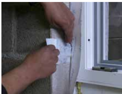
12. Apply Tyvek® Plastering tape to the window head and reveals taking care to seal and brackets.
