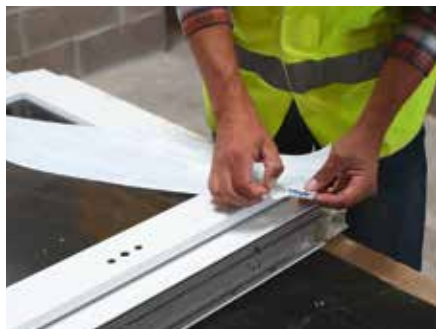
1. Using the 150mm Tyvek® Plastering Tape, start by removing the narrow release liner (20mm)
