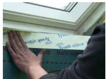
12. Seal tightly around window
