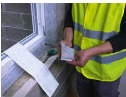
5. Fold in on itself to make a 3-sided corner
