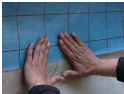
8. Fold DuPont™ AirGuard® AVCL onto primed surface
