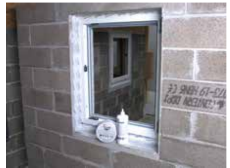
13. Repeat the process for the internal side of the frame and the gap is sealed!
