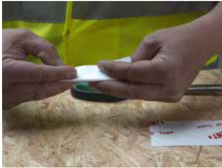
13. Fold DuPont™ AirGuard® Tape in half
