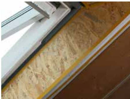
4. Tape should also be applied tight up to window/door frames
