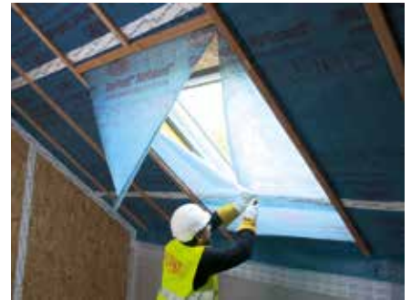
3. Cutting the vertical portion
