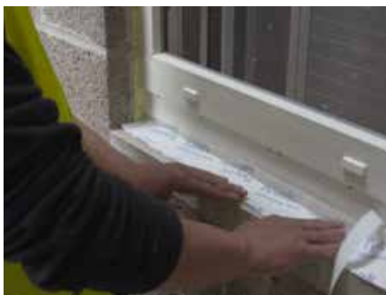
10. Press the tape firmly onto the primed surface
