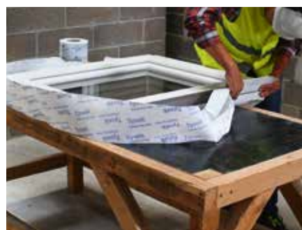
6. Repeat the same procedure as for the exterior side of the window. This time remove the large release liner of the tape (6 cm) and apply Tyvek® Plastering Tape to the window frame
