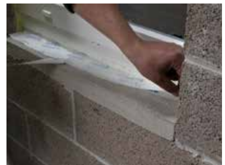
9. Starting at the cill, apply the exposed tape to the frame and remove the remaining backing strip
