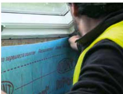
10. Position pre-cut AVCL and press against exposed tape adhesive applied earlier
