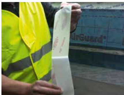
17. Remove release liner from DuPont™ AirGuard® Tape . . .
