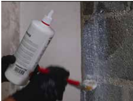
1. If the wall surfaces are chalky and need to be stabilised, apply Tyvek® primer
