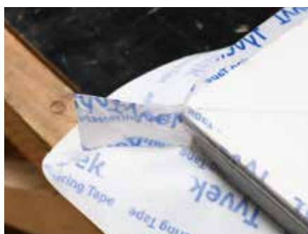
7. Form a loop on the corners: at least 1.5 x joint width - Repeat on all sides
