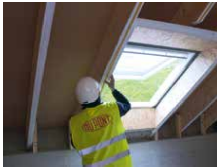
2. Apply tape to all facing surfaces . . .
