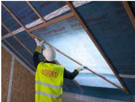
1. Cut a 'Y' into AVCL, using batten as a guide if preferred
