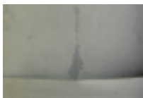
Indoor water damages
