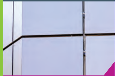
Typical Metal Façade
