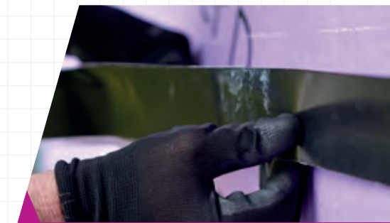
Weather Defence Joint Tape being applied
