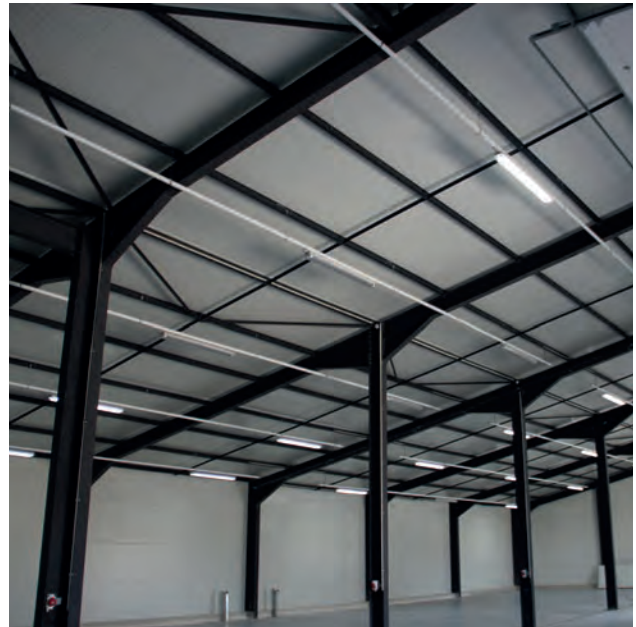
Vineyard storage building made in Jl Roof PIR
