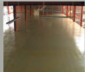
8. Floor completed in double quick time
