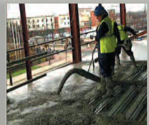
4. Mixture spread onto deck
