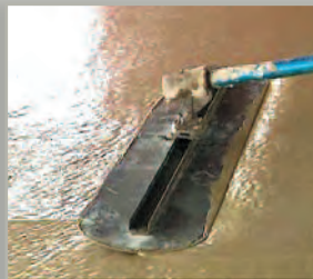
7. Floating provides a smooth finish
