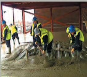
5. No mesh means no tripping hazard
