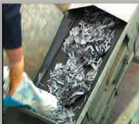
1. Steel fibres added to hopper
