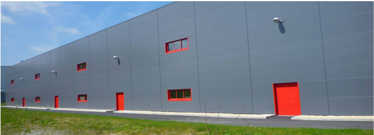
JI Vulcasteel Wall 1000SF used in an industrial project.
