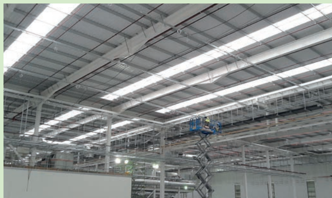
Project: Rolls Royce Advanced Blade Casting Facility Location: Rotherham Product: Zenon Curve & Evolution Liner
