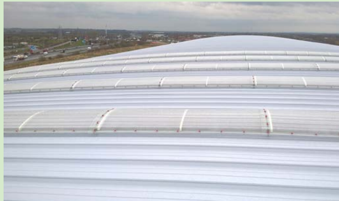
Project: Cornerstone Distribution Centre Location: Warrington Product: Zenon Arc & Pro Liner
