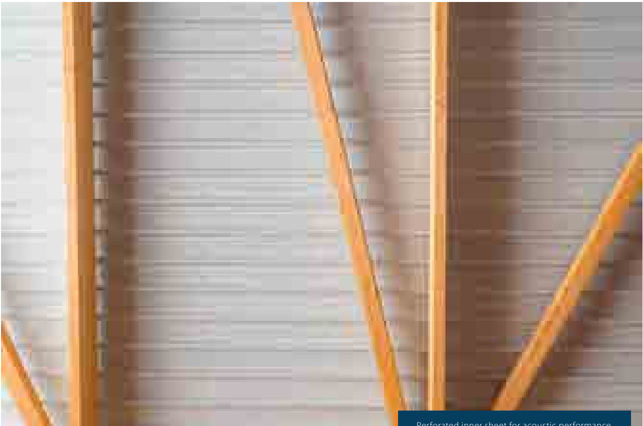
Perforated inner sheet for acoustic performance.
