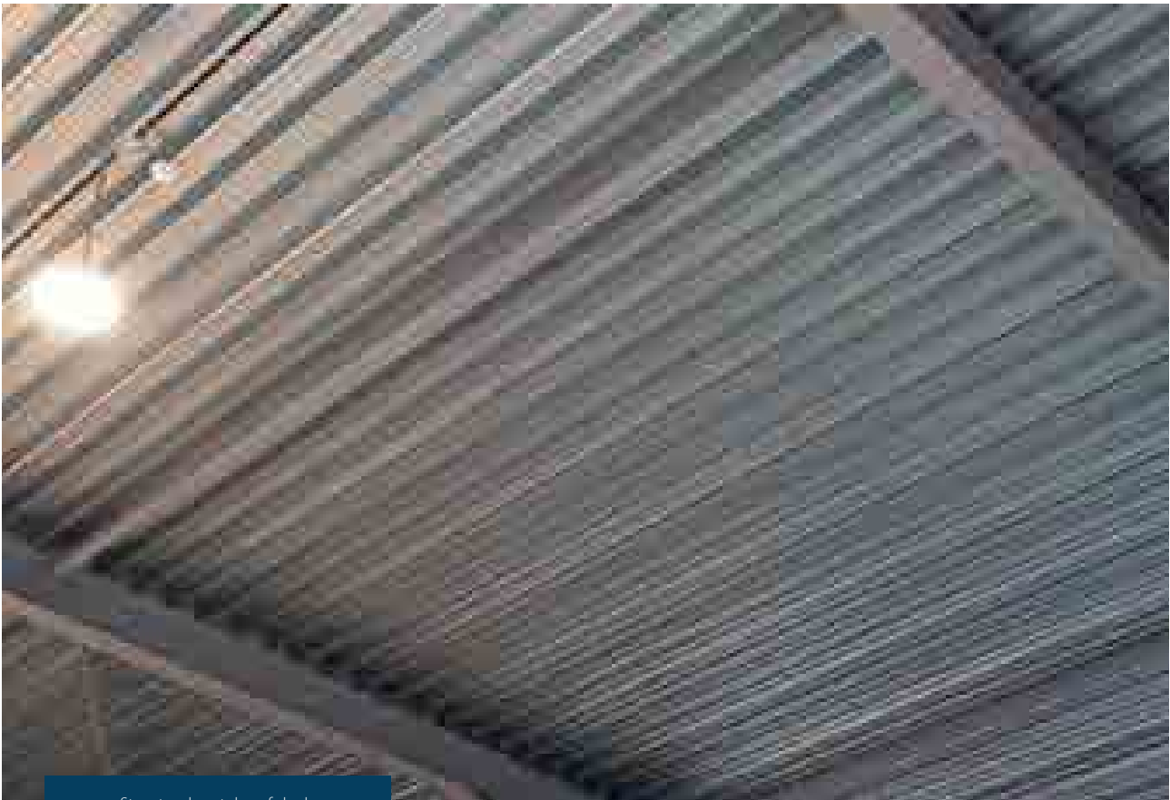
Structural metal roof deck.
